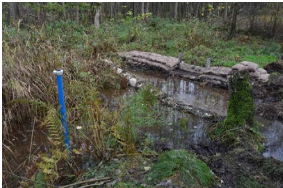
Dams implemented in the Deutener Moor to store rain water
