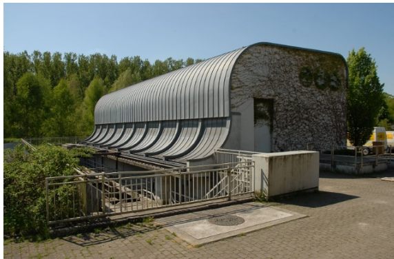
Pumping station Hammbach, pumping the creek over the Lippe-dike
