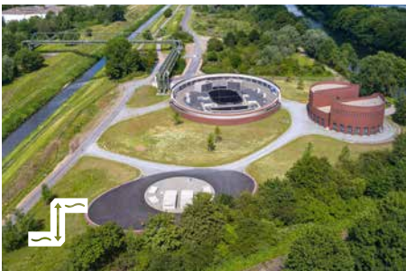
Gelsenkirchen pumping station
