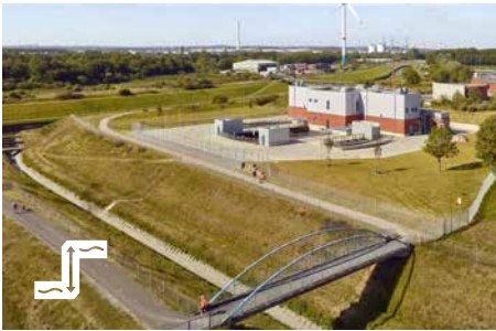
Bottrop pumping station
