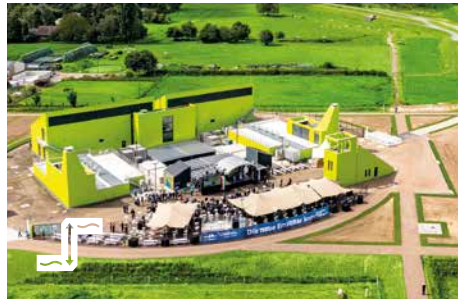
Oberhausen pumping station
