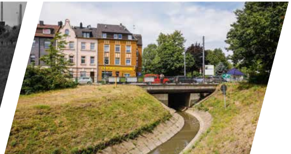
Wastewater flowing outside the front door
