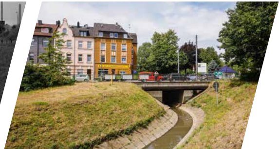
Wastewater flowing outside the front door
