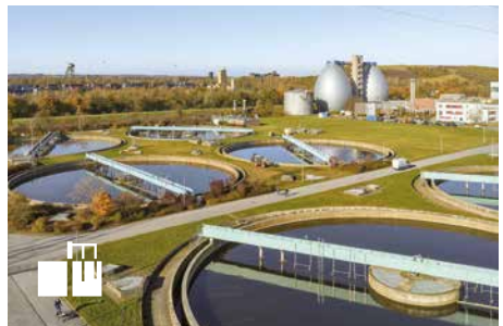
Dortmund-Deusen wastewater treatment plant
