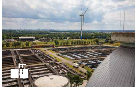
Bottrop wastewater treatment plant
