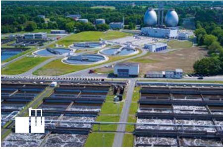
Emschermündung wastewater treatment plant in Dinslaken
