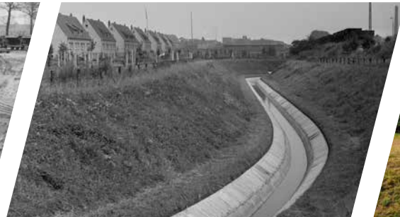
Open, concrete-lined wastewater channels
