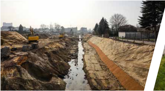
Ecological improvement of the Hellbach system in Recklinghausen
