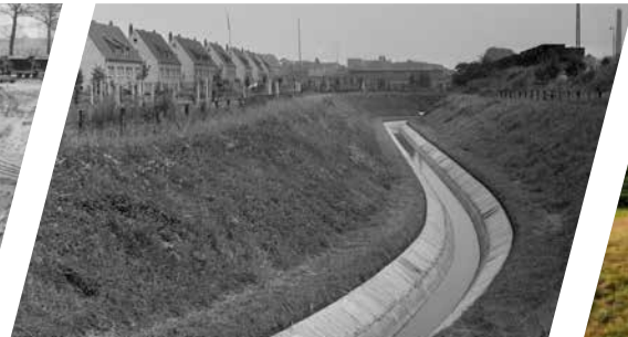
Open, concrete-lined wastewater channels
